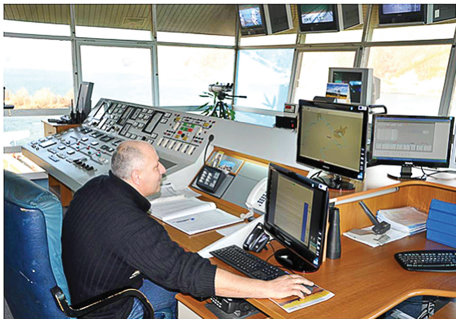
Figure 93. Control tower of the Đerdap 1 hydropower plant
